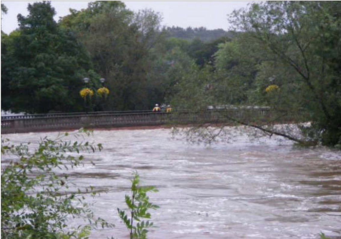
Figure 2-4: Oldgate Bridge in September 2008
